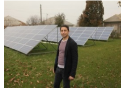
Photovoltaic equipment producer Moldova
